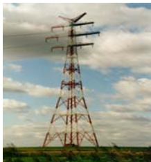
Pylon „Elbekreuzung" with a warning paint, height: 228 metres.
